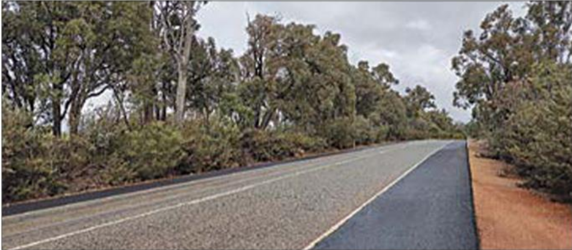
Low-cost sealed shoulders on Toodyay Road.
