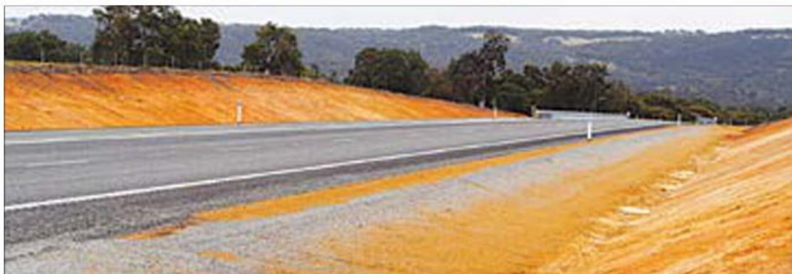
Grand engineering at Jingaling Brook but at what cost.
