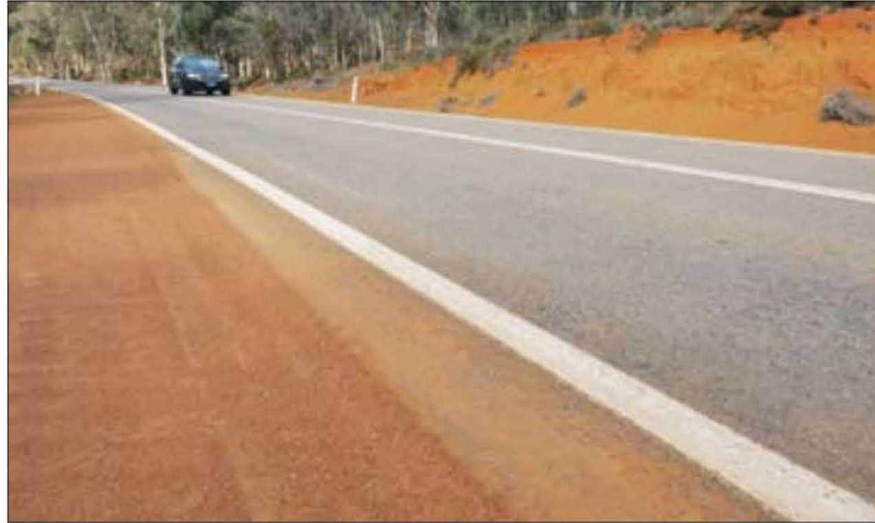
Recently repaired road edges on Toodyay Road.
